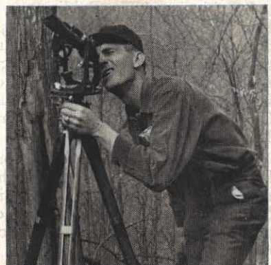
Robert Weddle, Pikeville district distribution engineer, takes a reading during the survey of the David to Falcon 44 kv line. Construction on the line started last month.
