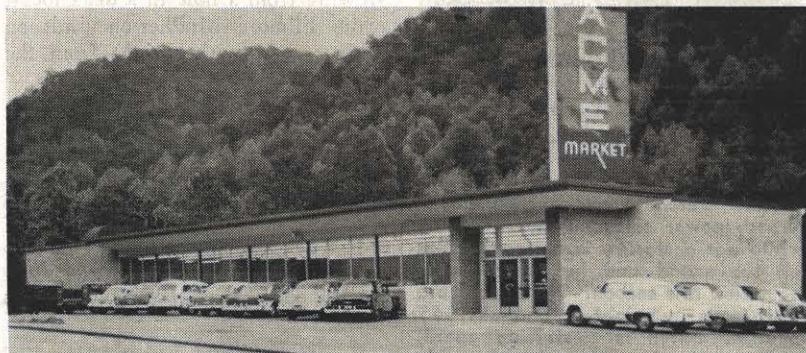
LEFT: First supermarket in the AGE System to use the heat pump for year-round air conditioning is this new Acme Market in Welch. The opening on September 29-October 1 climaxed completion of the all-electric building which replaced the market gutted by fire in March. RIGHT: Robert Porter, market manager at left, looks over a heat pump unit with Otho J. Bragg, Welch district commercial sales representative. An important point about the heat pump and the market was pointed out by Sidney Peery, Acme president, when he said, "While we are using all-electric equipment, we are also using coal—about the equivalent of 200 tons per year, coal by wire."
