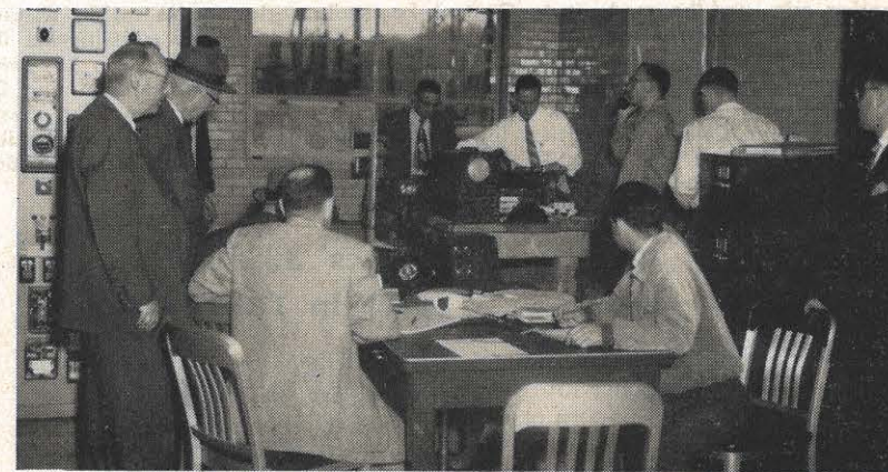
This is the inside of the control building during the oil circuit breaker tests. Instrument in the middle is a magnetic oscillograph.
