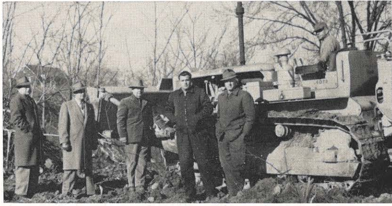
Present at the groundbreaking for the new Pearisburg office were, from left: W. J. Gillespie, Jr., Bluefield district manager; G. L. Poythress, engineer-inspector; L. L. Trinkle, contractor; E. L. Quisenberry, Pearisburg town manager; and R. A. Dobyms, contractor.
