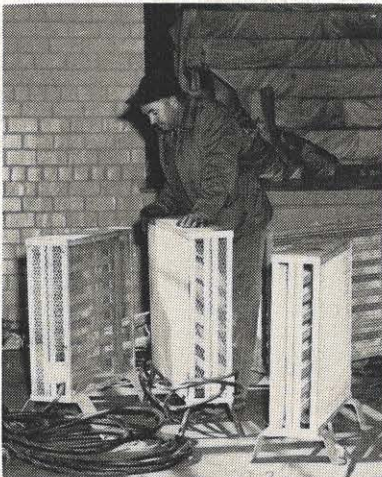
D. R. Whittaker, area supervisor, inspects some of the electric heaters brought to the Pearisburg Grade School.
