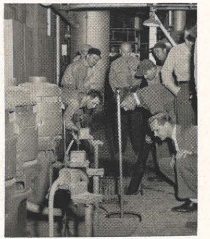
Observers watch closely as the foam fire protection system at Philip Sporn plant is run through a test.
