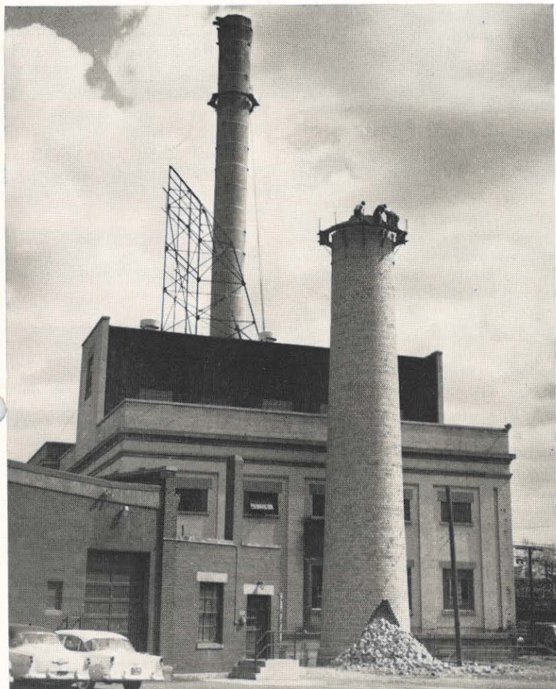
The two stacks atop the Walnut Avenue steam plant are disappearing from Roanoke's skyline. The brick stack at right went first when workmen chipped brick off and discarded it down the stack shaft. The stack was 8½ feet in diameter at the top and twice as large at the base.
