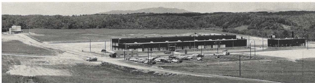
This is a general view of the Babcock & Wilcox Company nuclear facilities plant near Lynchburg. Fuel element fabrication building, gate house and steam plant are in foreground. At extreme left is experimental facility, where tests and experiments with nuclear reactor components will be conducted.
