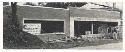
Completion is near on the new Pearisburg office building of the Bluefield district. The brick work is finished, the roof is complete and the interior job has begun. Four heat pumps will heat and cool the building, which will be completed in October.
