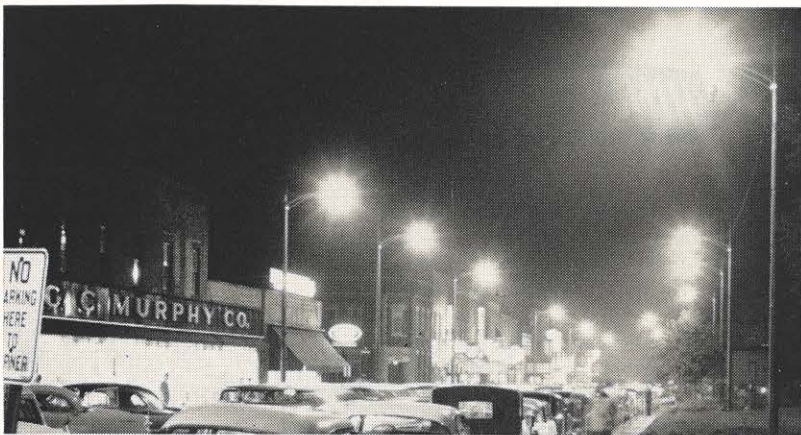
A good example of how a modern street lighting system can help a town in many ways is South Charleston in the Charleston District. This is 7th Avenue, one of the town's streets involved in a lighting program just completed by Appalachian. Besides helping improve the town's appearance, the lighting system will cut down on traffic accidents and crime, according to town officials. Fifty street lights were installed in this project, as well as new lines, transformers and other related equipment. The cost to the company for this project was $20,100. And as an indication of how towns are realizing the importance of street lighting, the South Charleston citizenry held special ceremonies when they cut on their new street light system.
