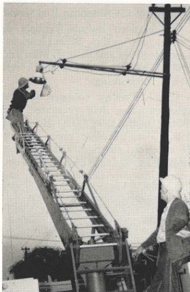
Following their regular schedule of street light replacement and cleaning are two Roanoke employees. J. M. Brown, street light attendant, is cleaning the fixture while J. L. Ferris, station man, observes.
