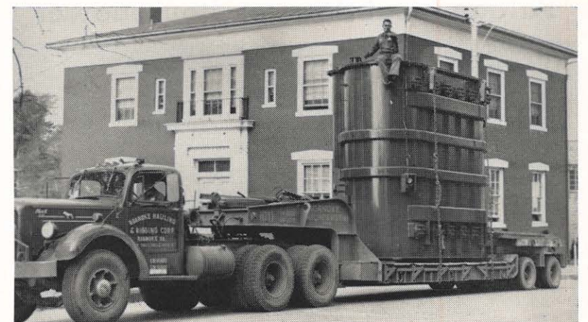
This 7,500 Kva transformer caused quite a bit of excitement when it was transported through Christiansburg recently. It was taken from a railroad sidetrack at Cambria through the town to the South Christiansburg station of the Pulaski district, where it will be installed. Several telephone lines had to be lifted out of the way by the man seated on the transformer. Addition of the transformer is just part of an expansion program planned at the station. Other work includes two oil circuit breakers, a bus regulator and construction of new 12,000 volt feeder circuits. Work will be completed next year.
