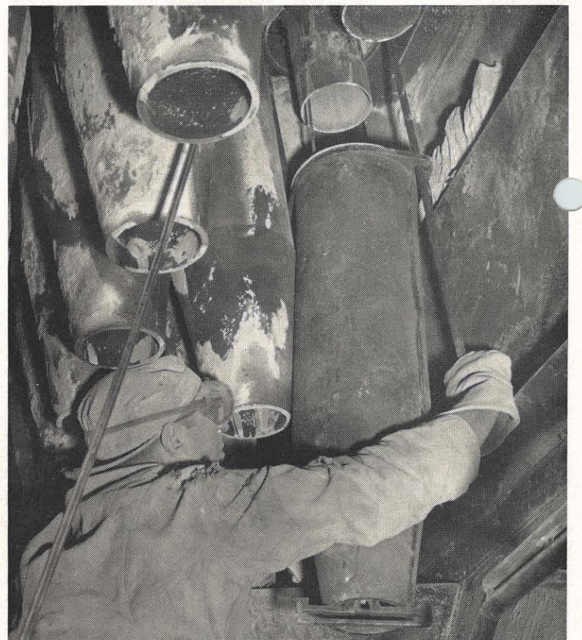
Standing below a pattern of tubes, C. C. Murrill helps in the completion of replacing a tube. With the aid of guide rods, plus the lifting cable, he is pulling the tube up into position inside boiler No. 2 at Kanawha River plant. These tubes are part of the process which prevents a high percentage of fly ash from being discharged from the plant stacks.
