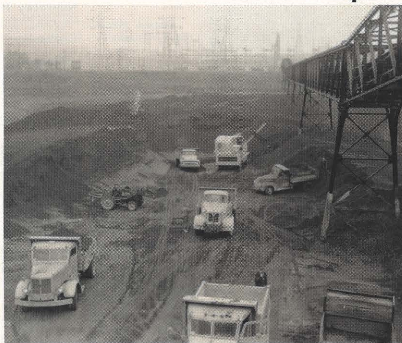
Under the giant coal conveyor at Philip Sporn plant six trucks are being loaded with fly ash and cinders. This plant waste product will be used on highways, roads and many other places in surrounding communities.
