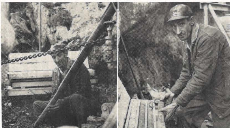
A driller of the Cunningham Core Drilling and Grouting Corporation of Salem removes the core from the barrel at left. At right, he puts it in a core box which holds 16 feet of core. These cores are inspected by a geologist who identifies the various changes in the rock and records the changes so that a map of the underground rock structure can be prepared.
