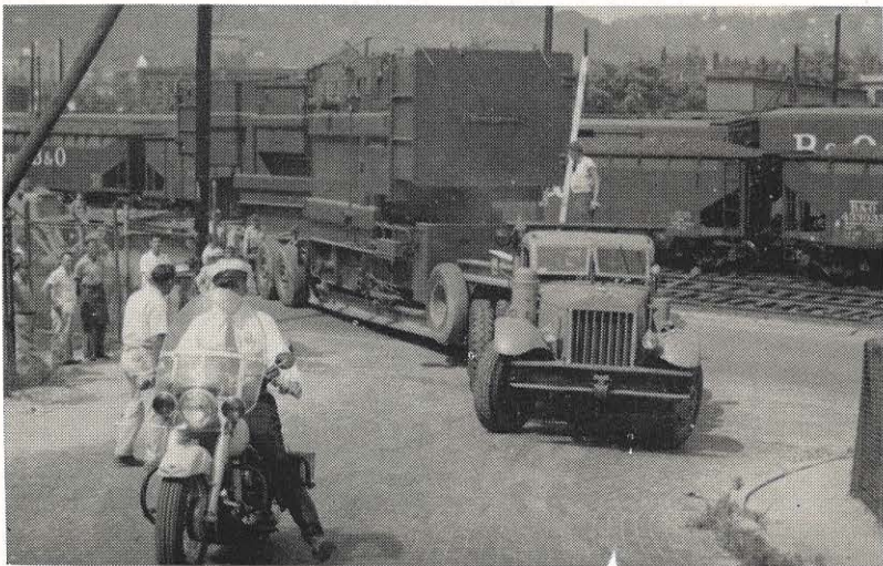
Patrolman Wayne Summerfield of the Charleston City Police prepares to clear the way as one of two giant transformers begins its journey to the site of the new Capitol Hill transmission station.
