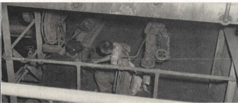
master maintenance man, are making routine repairs on an evaporator. RIGHT: Paul Stewart, maintenance man, and Glen Rouch, helper, make emergency repairs on a sootblower so it can be returned to service in time for the next day's load.
