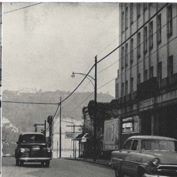
the cleaner look the city now has. Most of the cross-arms were removed during the project, which was begun in 1949 and cost almost $2-million. The conversion program involved the entire city.
