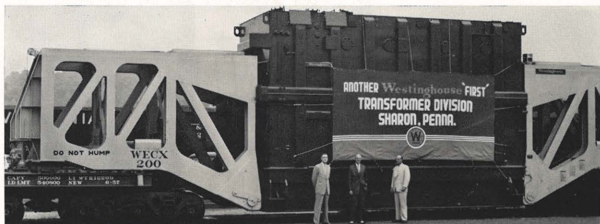
Headed for Ohio Power's Kammer plant now under construction at Foster, W. Va. is this giant 330,000-volt transformer, shown at a stop-over in Huntington. Inspecting the transformer and its unique railroad car are from left: Austin Neal, Huntington division supervising engineer; Hugh Stillman, division manager; and Julian
