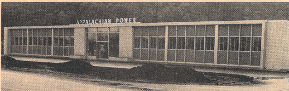
Over 1,000 persons attended the open house held recently at the new Point Pleasant office service building. The front of the building features white enameled brick with porcelain paneling. The 160 by 75-foot building is of split level design.
