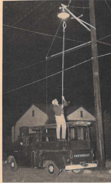
James E. Ford, Kingsport general serviceman, changes a residential street light during a service patrol at night.
