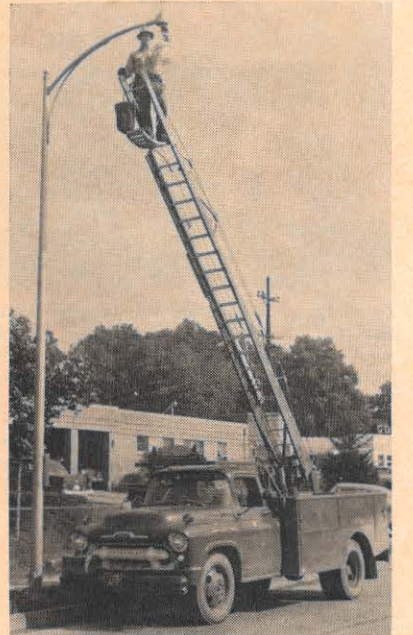
A modern lamplighter, James D. Spivey, Kingsport station man, replaces a whiteway lamp using a hydraulic lift ladder truck.
