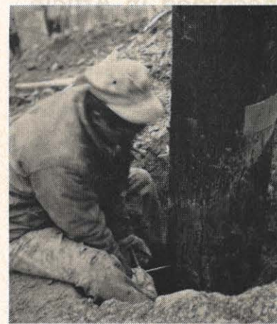
A pole "doctor" of the Muncy Pole-Treat Corporation tests for interior decay before injecting this Williamson district pole with a preservative solution. After the pole was "shot," tar was applied and the dirt replaced around the base.
