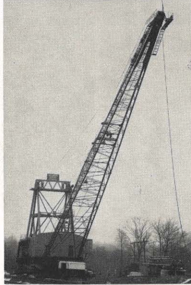
This giant is a 15-yard Marion drag line, and with the help of two Beckley employees, it was recently installed at the Quinwood operation of the Quinwood Mining Company. Henry T. Hutcheson and Mason T. Wood, power sales engineers, helped install a 700 hp synchronous motor on the drag line, which will drive three generators to provide power for the machine. This machine will be used in stripping operations to recover additional coal from contours already stripped. It is large enough to work a wall 100 feet high, and will deposit dirt on a spoil bank out of the way of the coal to be recovered.
