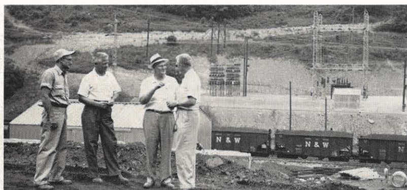
Discussing conversion work at the site of the new Clinchfield meter station in the Abingdon district are from left: L. F. Valley, Russell County area supervisor; R. M. Bondurant, district superintendent; C. W. Johnson, meter supervisor; and L. C. Angle, Jr., district commercial manager.
