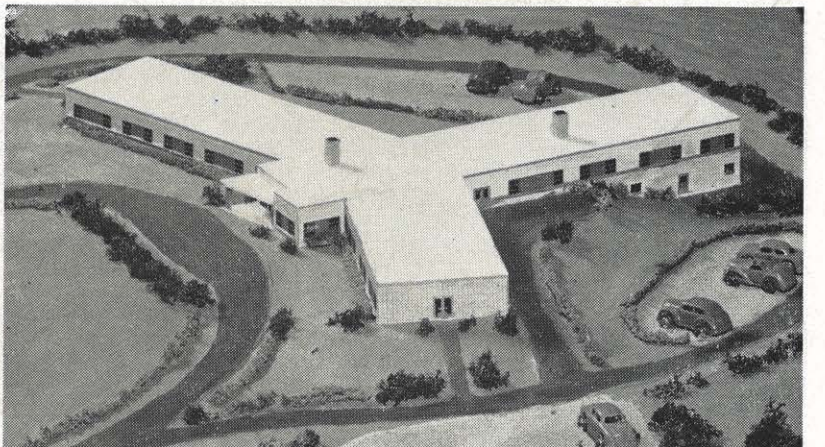
Groundbreaking ceremonies were held recently in Point Pleasant as a kick-off for construction of the 40-bed Mason County hospital. Shown here is the architect's model of the $588,000 structure. The hospital features individual window heat pump units for each room and electric water heating and sterilizing equipment.
