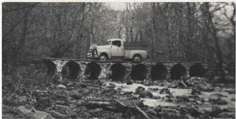
This bridge may end a 100-year-old problem in the Snidow family. S. S. Snidow, Roanoke district auto repairman, recently completed the structure which leads to his farm in Giles County. Because rains can make the creek violent, previous attempts to put in a bridge have met with failure.
