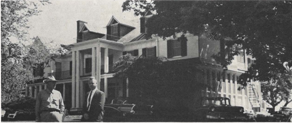
Pausing in the front yard of his mansion is J. E. Covington, left. With him is Jack M. Burnett, Fieldale district commercial manager. Built by slave labor, the mansion has been remodeled for all-electric living.
