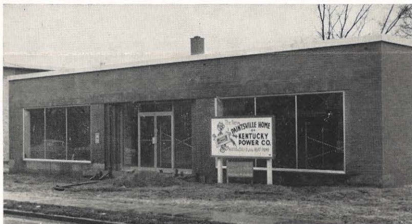
The Paintsville office building has donned its exterior as construction nears 75 percent completion. Located in Kentucky Power's Pikeville district, the structure is scheduled to be completed by late spring. The heat pumps have been installed and are in operation. Plastering of inside partitions and walls has been completed, but floors and ceilings are unfinished.
