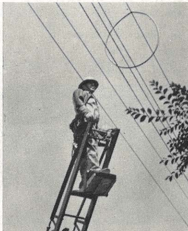
Charles E. Howell, Bluefield meter serviceman, prepares to remove the mysterious hula hoop circling a 6,900-volt hot wire. How did it get there? Nobody knows.
