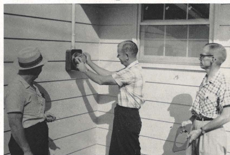
Fred LaRue, area sales representative, left, and M. C. Simpson, commercial manager, right, watch as J. W. Bolton, meter supervisor, installs a meter on Kingsport's 2,500th electrically heated home.
