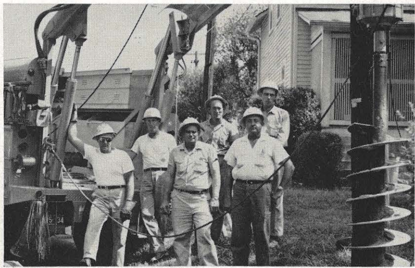
Liew Osborne and his Ashland district crew pose proudly with their new hydraulically-equipped truck, first one in use in our companies. The truck has a jack, boom, winch, and pole and anchor hole digger, all hydraulically operated. Manning the new truck are, from left, Ray Adkins, lineman; Mason Gallaher, lineman; George Price, serviceman; Calvin Burnett, truck driver; Liew Osborne, foreman, and Russell Scaggs, groundman.
