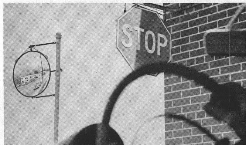
Ingenious installation of a mirror has solved a serious traffic problem at the Bluefield district's Pearisburg office parking lot entrance. Previously, drivers emerging from the lot could not see traffic coming from the left. Now a convex, 26-inch mirror mounted on a pole enables street traffic and parking lot traffic to see each other coming. The Pearisburg people, not willing to lose an opportunity, used the reverse of the mirror as sign board for the cheerful invitation: "Live Better Electrically."
