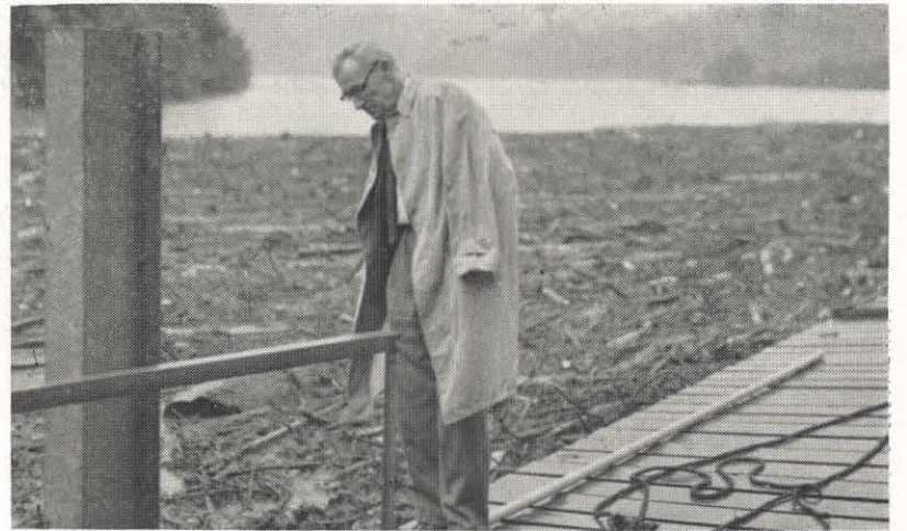
Heavy rains and floodwaters, brought by Hurricane Gracie, lashed parts of Appalachian territory, leaving some damage in their wake. Here, A. D. Clark, Pulaski district superintendent, watches as logs and trash are being worked through Buck hydro plant's sluice gate. Note the large quantity of debris in the background. Mr. Clark reports that more water passed through the spillways at Byllesby and Buck hydros than at any other time since 1949. Elsewhere, small streams and rivers overflowed their banks, doing some damage, while winds toppled trees and limbs into lines.
