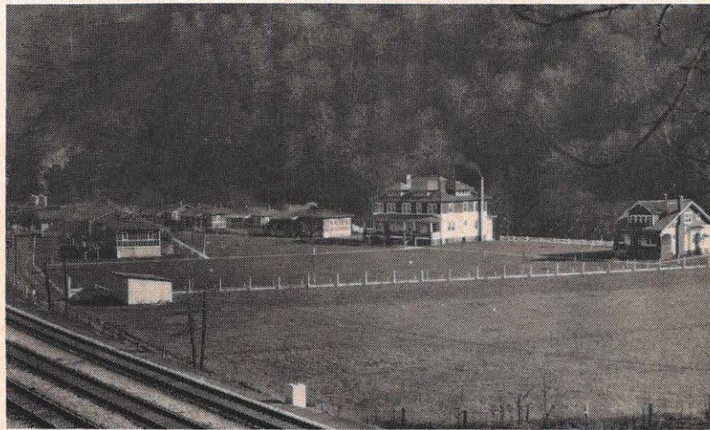
Another power company landmark is disappearing as the last of this camp at Sprigg, W. Va., is being razed. The large building, now occupied by the Tug Valley Country Club, and the house at the right are all that remain, but they too are being torn down to make way for a new, modern clubhouse. This picture of the camp, which was built in 1916, was taken October 3, 1931, and shows the 12 camp houses and clubhouse. In these houses lived the employees who helped operate the old Sprigg power plant, and those who helped construct and maintain lines in the area.
