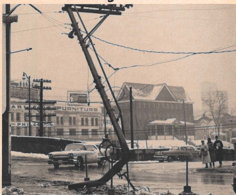
Appalachian's power poles in Bluefield are tough. This one, a steel pole, was in the way of a skidding Greyhound bus not long ago. The impact knocked out circuit breakers and interrupted service to some customers briefly.
