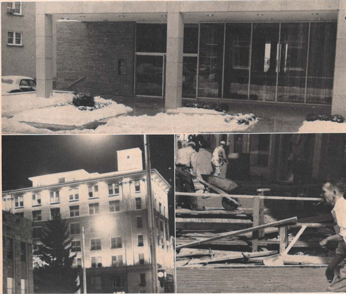
TOP: Electric heat cable in action de-ices and de-snows the sidewalk in front of Beckley's Bank of Raleigh. BOTTOM LEFT: The Raleigh County Bank, which has also installed the sidewalk cable, highlights the skyline with its
