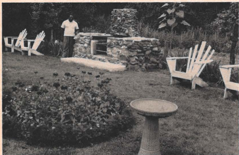
Dunbar Hill poses beside the barbecue pit and fireplace he built in his yard. It took 375 stones of assorted sizes, 18 cinder blocks and three bags of cement, plus 80 hours of work to do the job. Mr. Hill is janitor in the Roanoke district.
