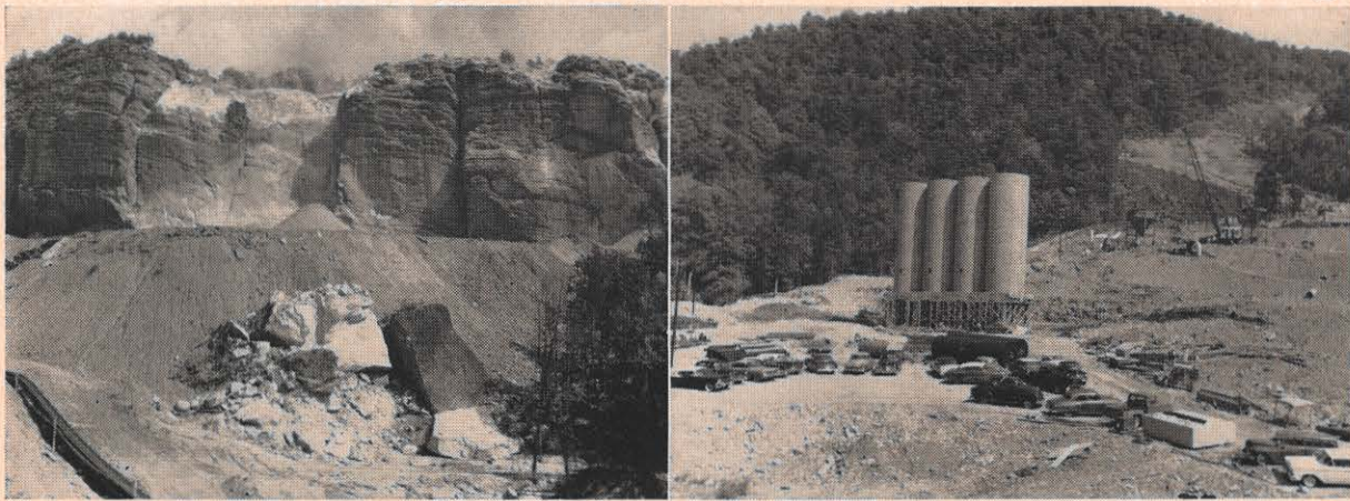
Operations at eastern Kentucky's biggest new industry are beginning. It's the quarrying and crushing work of the Silica Corporation of America in Pike County. In the picture at left, a conveyor will carry the quarried
