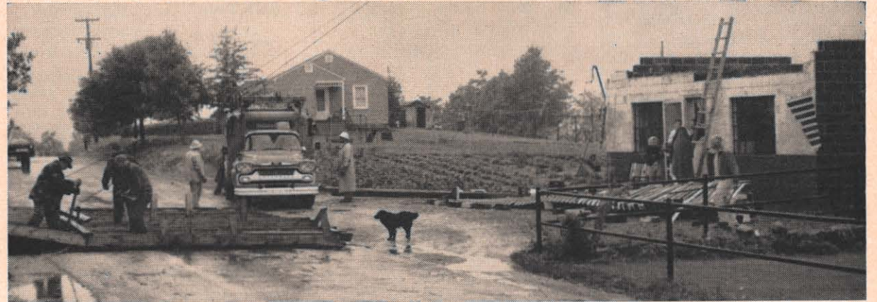
Wind lifted the roof from this store in the Oak Hill area in the middle background, and the distribution line carried and placed it in the road. Note the Appalachian crew to the ground by the roof.
