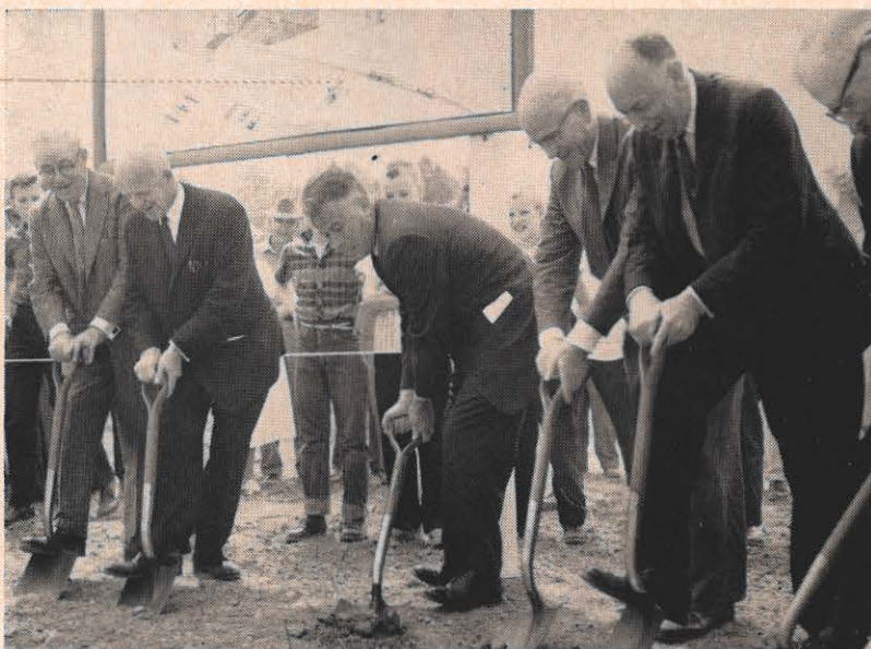
Digging with vigor despite the 90-degree heat at the Big Sandy plant groundbreaking were, from left, Boyd County Judge E. K. Rose; Kentucky Power Vice President and General Manager F. M. Baker; Governor Bert T. Combs; AEP President Philip Sporn; Lt. Gov. Wilson Wyatt and, partially shown at right, Kentucky Public Service Commission Chairman J. David Francis and Lawrence County Judge Nile Ball.
