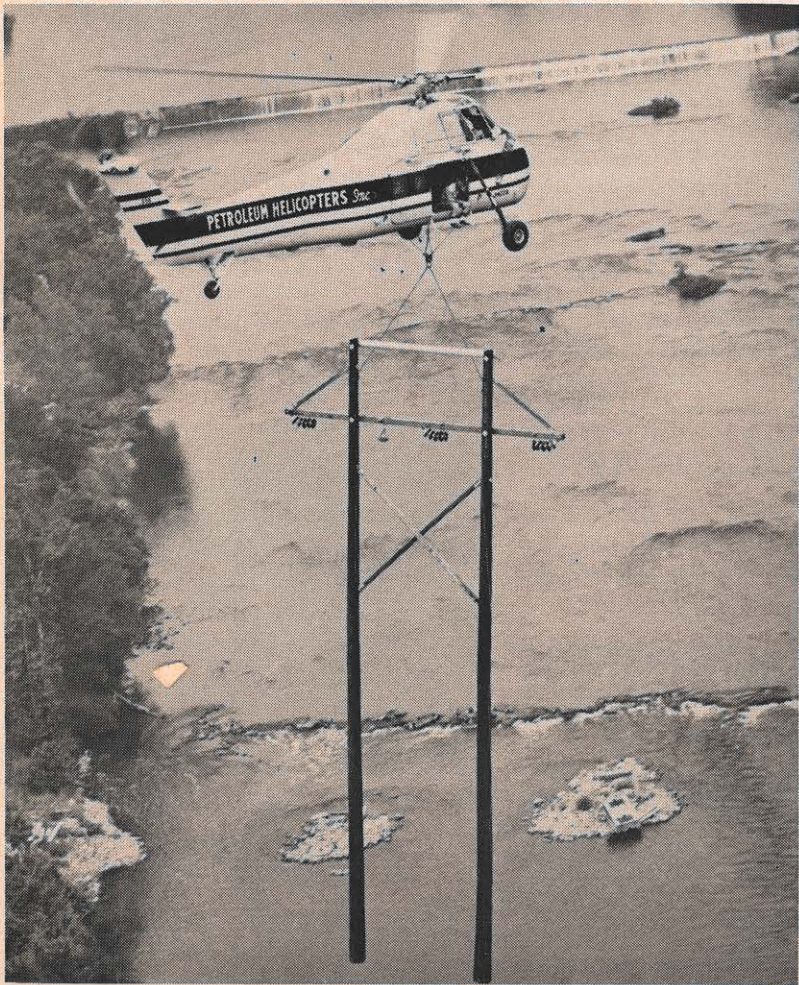
The James River forms a scenic background for the helicopter as it hauls an H-frame structure on the South Lynchburg-Big Island line. Out of the picture to the left is the Owens-Illinois Glass Company plant. Photo courtesy Sikorsky Aircraft.
