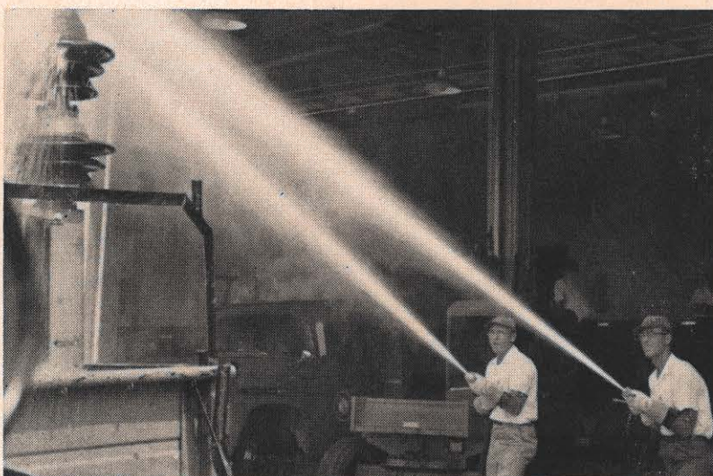
During the public showing of the Bluefield service building, Fred Combs, left, and K. A. Hayes of the system transmission department, demonstrate the high-pressure washing of insulators. Water pressure from the hose is 750 pounds per square inch.
