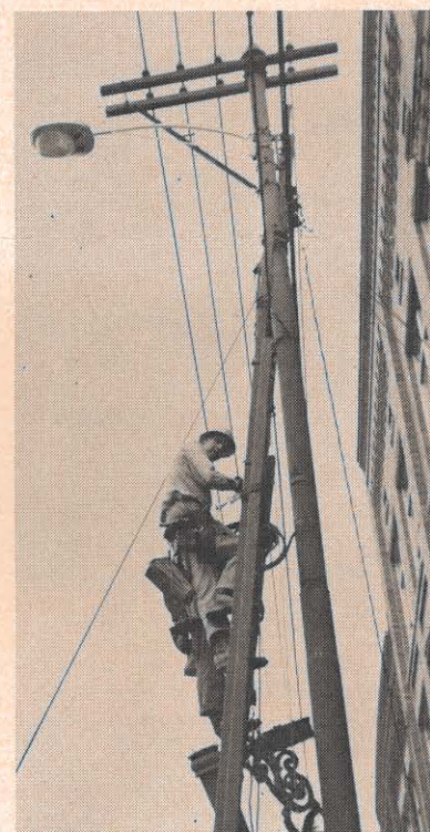
A pedestrian's eye view of street light work illustrates a new lighting project in Charleston. Slim Bailey and Danny Acela (behind Slim) remove 4000 and 6000 lumen lights, installed in 1930, in the Washington Street section of Charleston. Taking their place are 21,000 lumen mercury vapor lights, like the one above the men, each individually controlled by sun switches. Here 24 old lamps were replaced by 27 new ones. In Kanawha City, along its whiteway, 21 more of the new lights were also installed.
