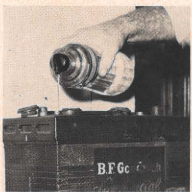
Garlin E. Hill, Bluefield district stationman, discovered a better way to do his job. He found that the rubber syringes he uses to fill substation batteries corroded from the acid. A used quart ink bottle with a pouring spout does it better.
