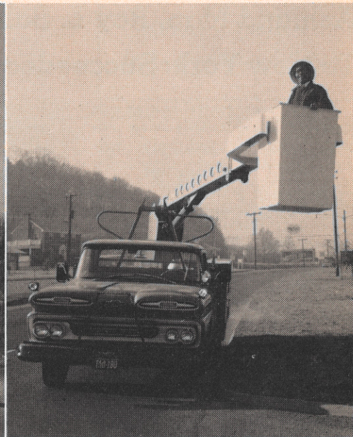
quite in position for replacement. Both are district street light attendants. At right, Mr. Pullen is shown after he has replaced a lamp and is lowering the bucket into the cradle on the truck, preparatory to being driven to the next street light.
