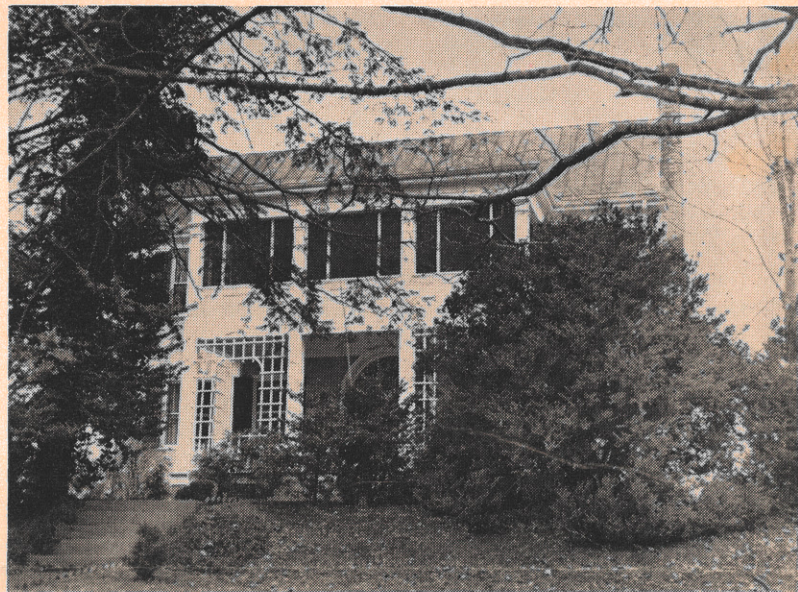
Two hundred thirty years old, this house has been modernized and now has electric heat. The Kingsport home evolved from a two-story log cabin.
