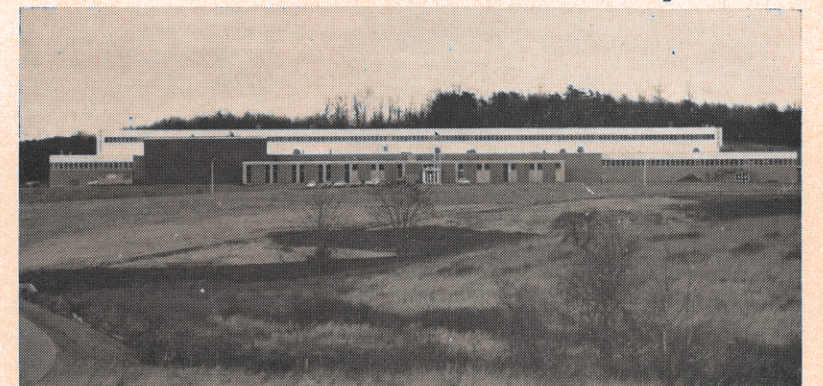
The H. K. Porter Company will soon begin full-scale operation in its new plant and office in Lynchburg. Operations should begin sometime in February, according to company spokesmen, and office quarters are already in use. The plant was built by Lynchburg Area Development Corporation for lease to Porter, and it represents the first time that pre-stressed concrete has been used in such a large building in the area.
