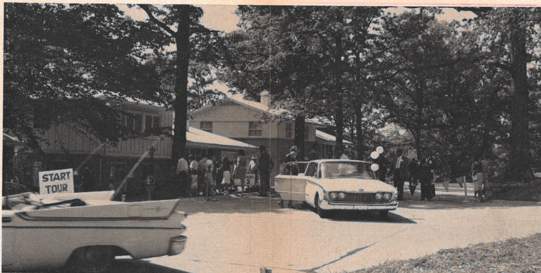
A highlight of the year in commercial activities was the announcement, and construction start, on the Arlington Park subdivision in Huntington. The subdivision will have 180 Gold Medallion Homes, and is the largest all-electric development in our companies. The homes range in price from $20,000 to $55,000. To date, 42 homes have been completed and 14 others are under construction. Fifty of this total have been sold, and of the 42 completed, 37 have been occupied.
