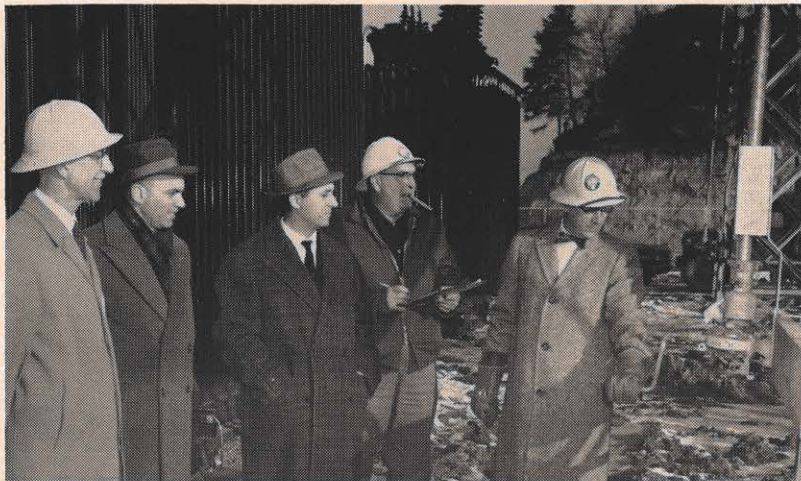
Energizing the South Neal station of the Huntington district were, from left: H. B. Hout, division station engineer; Loris Luciano, Montecatini (of Italy) development engineer; Dr. Carlo Vancini, plant manager for Novamont; V. L. Thacker, station supervisor; and S. R. Pritchard, district manager. Novamont is Montecatini's wholly-owned American subsidiary, and is building a plant at Neal in the Huntington district. The South Neal station will help supply the electricity for operation of the plant.
