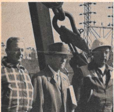
These three men were instrumental in the setting up, conducting and supervising of the anchor tests. They are from left: J. W. Engleby, Jr., system senior civil engineer; R. B. Sinclair, system civil engineer; and B. F. Cory, assistant construction manager for Hoosier Engineering Company.
