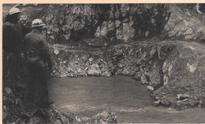
Checking survey control targets at Smith Mountain are Ralph Mudgett, civil engineer, and Jack Towler, a member of his crew, which also consists of Morris "Whitey" Barbour and Artis Barbour. The men are standing on the north side of the mountain and across the river can be seen part of the thrust block and keyways for the south side of the dam. At river's edge can be seen the cut made by the spillway and powerhouse area excavation.
