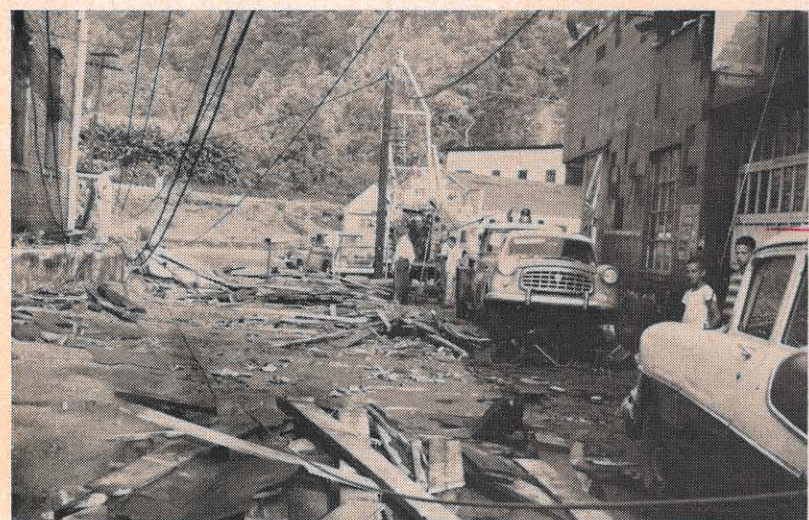
This scene was typical of the aftermath of the heavy storms that struck the Williamson district last month. Hardest hit was Matewan, where electric service was disrupted and heavy property damage was reported. Picture courtesy "Williamson Daily News".
