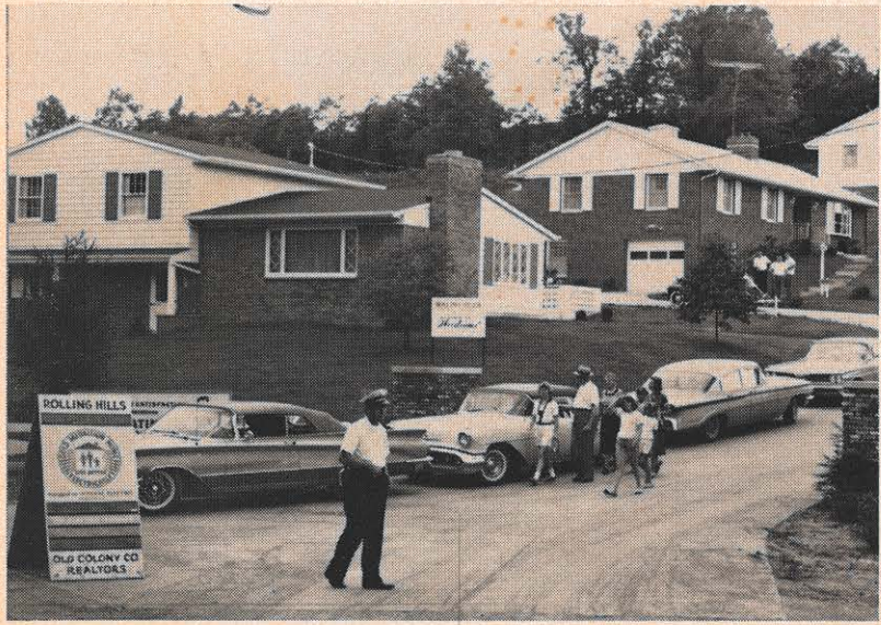
Three thousand people saw total-electric living close up during the open house held by the developers of Rolling Hills, Charleston's newest and largest Gold Medallion subdivision. Appalachian personnel explained all-electric living to the visitors who flocked in all week to see the heat pump-equipped homes.
