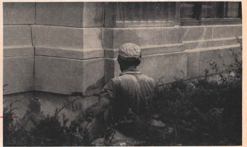
For the first time in more years than anyone likes to think about, the exterior of the Charleston Virginia Street office is undergoing a cleaning. Old mortar has been cleaned out and replaced and jet streams with sand feed have cleaned the building's surface. Note in this picture the contrast of the new look with the old.
