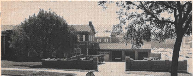
Seven hundred square feet of space have been added to the Kingsport Utilities' parking lot. This increases the lot's capacity from 20 vehicles to 32. The lot was originally completed in 1932.
