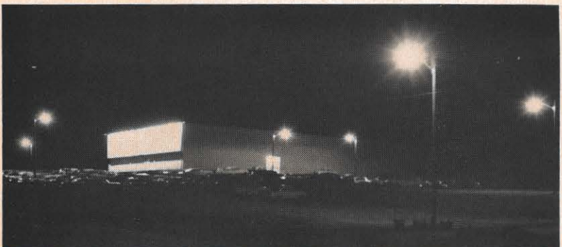
Happy Lanes has opened between Pearisburg and Narrows, providing 16 lanes and all-electric facilities. In addition, the modern bowling center has eight Dusk-to-Dawn lights ringing the parking area, six of which can be seen in this photo. The lanes are in the Bluefield district.
