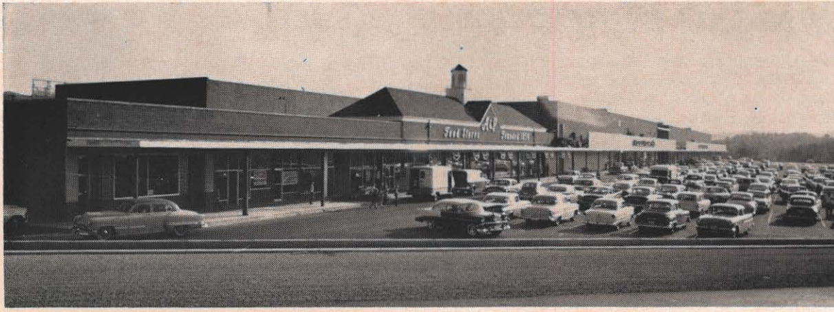
Towers, Roanoke's newest shopping center, is using more electricity than any other shopping center in Appalachian territory. Photo courtesy "Roanoke Times."
