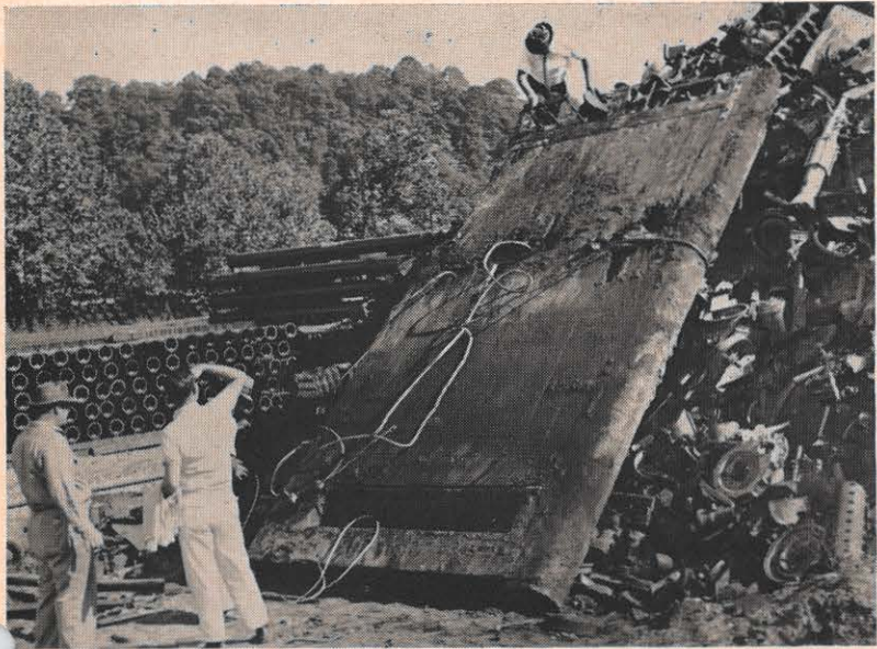
National Park Service men examine carefully the lock gate excavated from the rubble-filled lock of the old James River and Kanawha Canal in Lynchburg. Reconstructed gates copying these will be installed in a working lock of the old canal where the Blue Ridge Parkway crosses the James River at Big Island, Virginia. The sluice gate at the bottom allowed the water to flow into the lock before the gates were opened.
