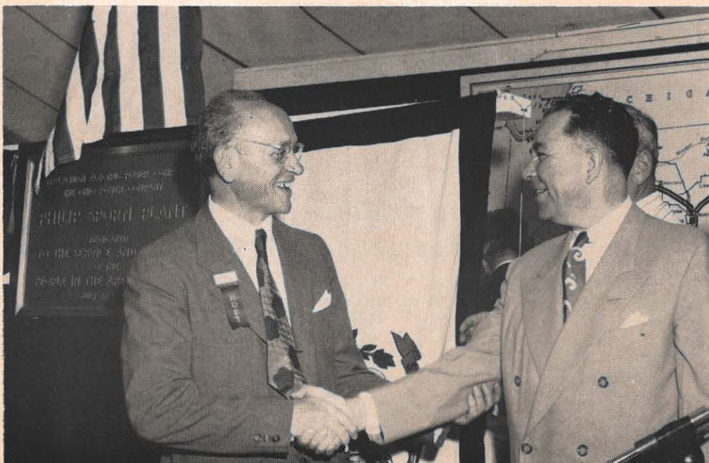
A singular tribute came to Mr. Sporn when the AEP directors named the Philip Sporn plant in his honor. Here, at the plant's dedication in 1950, West Virginia's then Governor O. L. Patterson congratulates the company president. This 1,100,000-kilowatt station, the System's largest, is jointly owned by Appalachian and Ohio Power.
