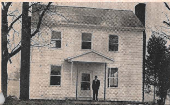
This home is the 1,000th electric heating job installed in the Lynchburg district. It is owned by P. M. Stinette, Clifford, Va., and is a conversion installation, using base-board units. J. F. Wilson, Jr., district heating and builder sales representative, stands on the porch.
