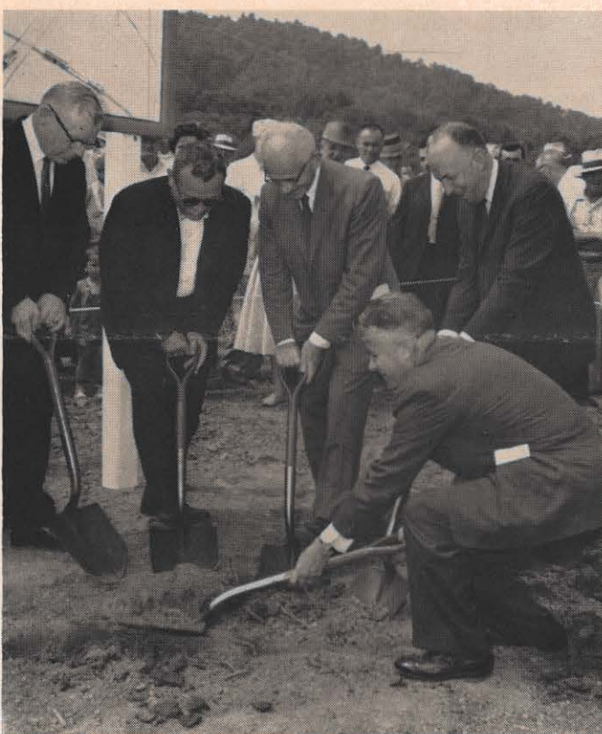
Kentucky Governor Bert Combs (foreground) shows 'em how as ground is broken for Kentucky Power Company's new Big Sandy Plant near Louisa, Ky., in 1960. That's President Sporn wielding the shovel in the middle.
