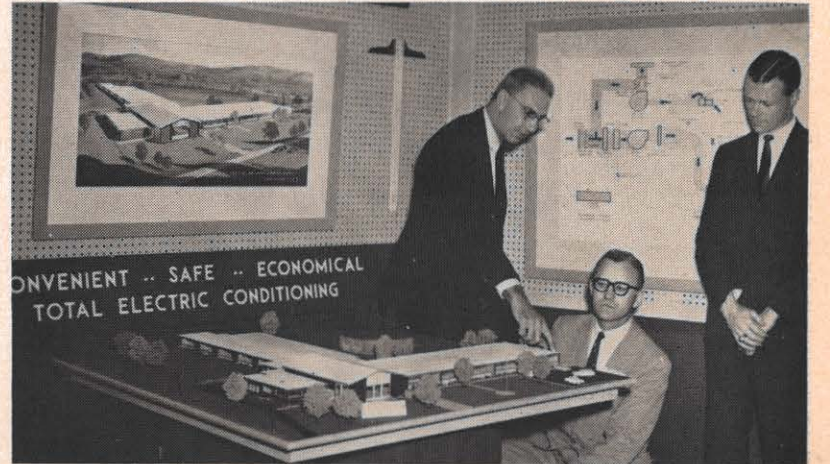
An exhibit featuring the Paul Munro Elementary School and its unique heating and ventilating system was a highlight of the biennial meeting of the Virginia Chapter of Architects, the Virginia Society of Professional Engineers and National Society of Professional Engineers. The exhibit was prepared by the Roanoke division of Appalachian. Shown in the picture are from left: J. Everett Fauber, Jr., architect for the school; Lewis D. Evans, Roanoke division heating engineer, and B. Gordon Watkins, Jr., associate of Wiley & Wilson, consulting engineers of Lynchburg, engineering firm for the school.
