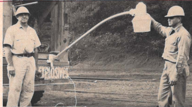
A new application of Dusk-to-Dawn lighting, and a new way of installing them are shown in these two pictures, above and right. Before a light can be installed it has to be assembled and wired; and since the arm of the light is bent, this can be an awkward task. The Tazewell line crew of the Bluefield district devised a simple system to do a better job; they installed a bolt stud in the back of the truck and the arm is hooked on. Smith Compton, groundman, and Joe Claytor have just finished one light. At right, lighting two levels of a Roanoke parking lot is a unique two lights-on-one pole installation. It was sold by T. C. Smith, Roanoke division dealer sales representative, who has sold 223 since April.
