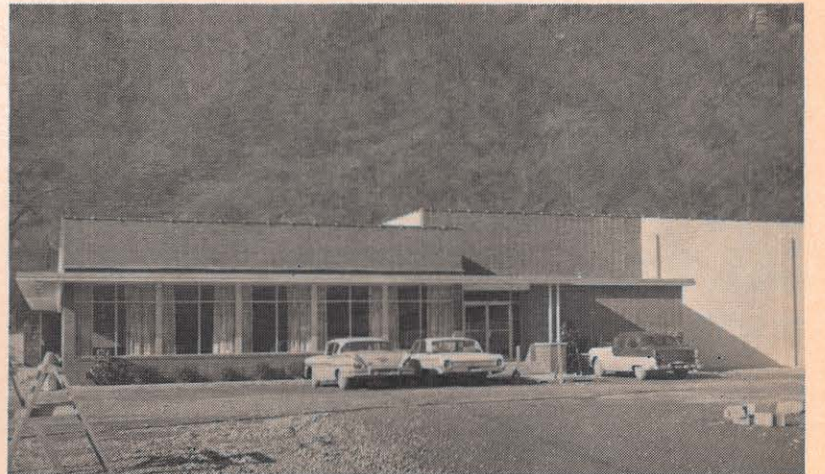
This is the first all-electric bowling establishment in the Pikeville district. It is heated and cooled by four ten-ton heat pumps, has a kitchen, dining room seating 300, nursery—and 16 bowling lanes.
