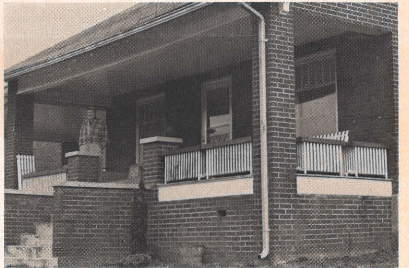
C. P. McClaugherty, a resident of Narrows, Virginia, has found a new use for old radiators. When he installed electric heat, he found himself with a number on hand. Solution: convert them to porch railings, and use the wooden covers for potted plants and flower boxes. He is a retired employee of the Virginia Department of Agriculture.
