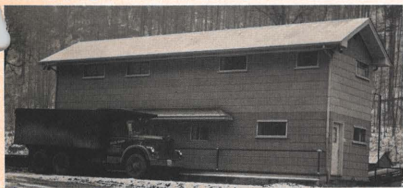
In the heart of the Welch coal fields sits this new, modern scale house, heated and cooled by Buchanan County's first commercial heat pump installation.
