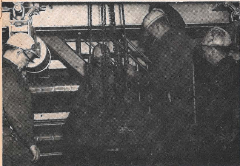
During a planned outage on Clinch River Unit 2 recently, cleaning turbine control valves, acid washing the boiler and cleaning the air preheaters were all completed. Here Lee A. Singleton, Perry E. Miller, James R. Trail and Clarence E. Browning replace the main stop valves.
