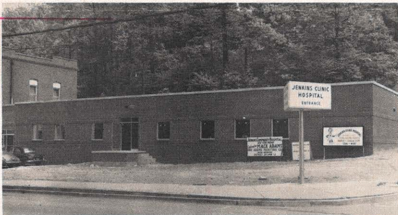
This is Jenkins Clinic Hospital, at Jenkins, in the Pikeville district. It is the first all-electric hospital in Kentucky. Completely fire-proof, it contains six nursery beds, 16 adult beds in semi-private rooms and six pediatrics beds. It has a connected load of 196 kw.
