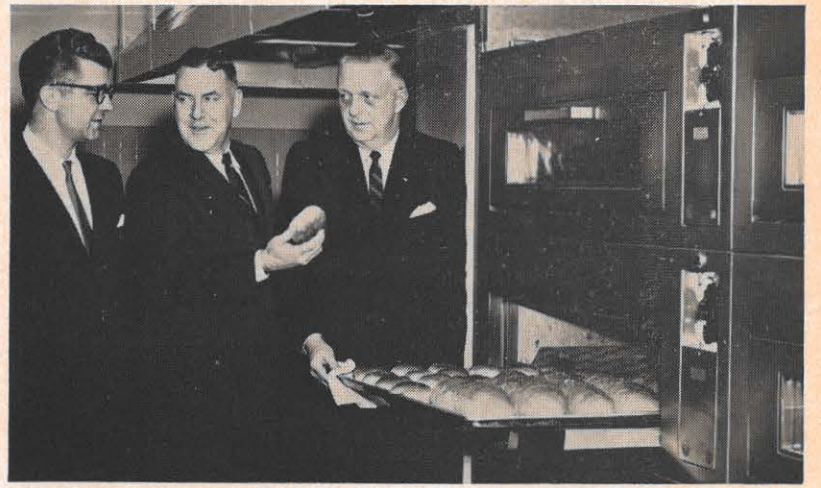
One of the newer total electric installations in Roanoke is Bailey's Cafeteria in the Crossroads Mall. Here C. W. Moore, Roanoke division commercial sales engineer, admires bread being turned out in an electric oven. At left is Rome Coffey, manager of the cafeteria, and at right is Fred Grim, vice president of the Ted Burton Company, cooking equipment dealer. This cafeteria was going to gas, but with Mr. Grim's help, it went total electric for a cooking load of 175 kw and 30 kw in heat pumps.
