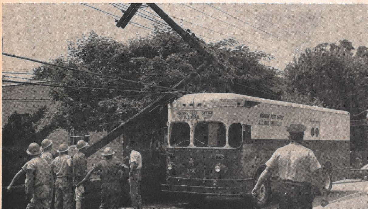
Service continued unabated, even though this mail truck broke a power pole in Pikeville at the sidewalk level and again halfway up. Here a Pikeville district crew prepares to replace the pole, which supports one
