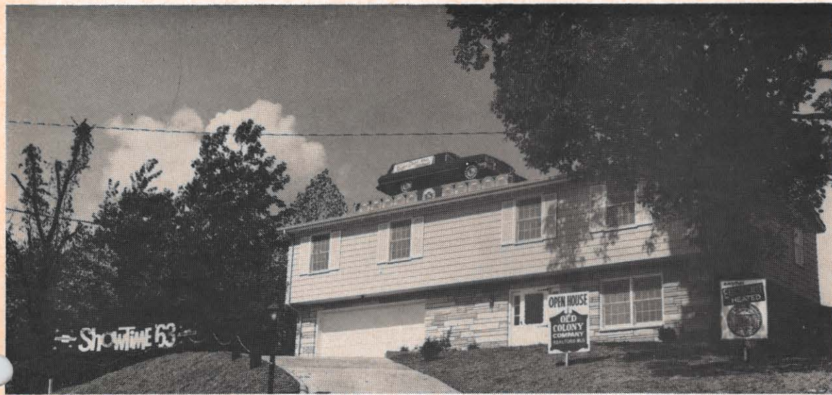
One kind of solution, though not recommended, to parking problems was offered during a recent Gold Medallion Home open house in Charleston. A new station wagon was hoisted to the roof to demonstrate the strength of truss construction. The two homes open to the public are in Rolling Hills; one is heated
