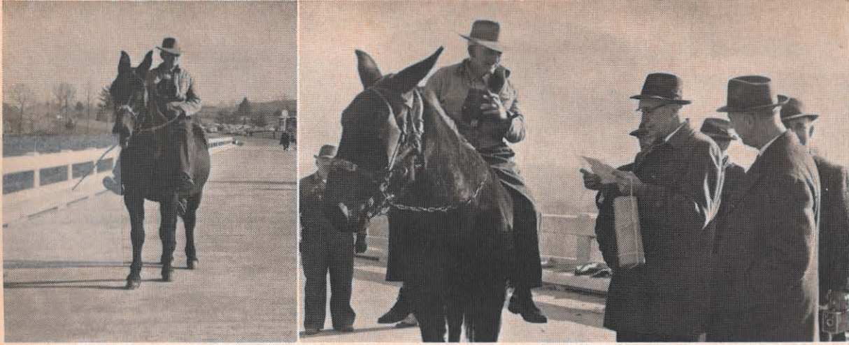
First official traffic across the Haleford Bridge, Jap Hundley and his mule, Jack, are shown at left close to the end of the 1,000-foot journey. At right, J. L. White, Roanoke division engineer, reads to Mr. Hundley a "Certificate of Primacy" as proof of his achievement. With Mr. White is Rev. H. L. Cooper, member of the Bedford County Board of Supervisors. It is the fourth Haleford Bridge Mr. Hundley has crossed.
