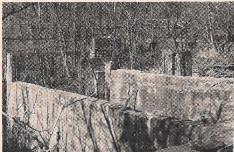
A few concrete piers and brush are all that is left of the Montgomery Electrical Company at Grayson, an early 20th Century predecessor of Appalachian.
