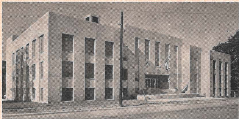
The Mason County Courthouse is the only one in Appalachian territory making use of heat pumps for heating and cooling.
