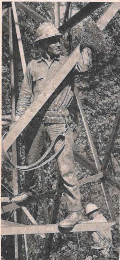
An experimental hand mitt was used during a painting job on a river crossing tower in Point Pleasant not long ago. Manufacturers claim the mitt is quicker, easier than a brush. That's R. L. Barrette, lineman, using the mitt.
