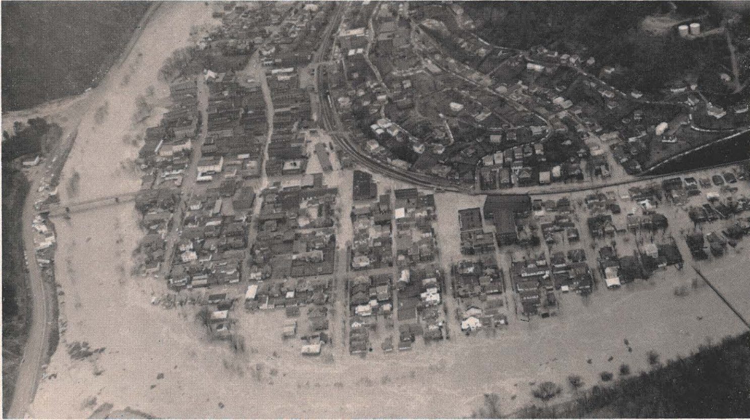
The record flood that hit Pikeville is shown swirling through the Kentucky city. Most of the water is from the Levisa Fork of the Big Sandy River. Photo courtesy Huntington Publishing Company.
