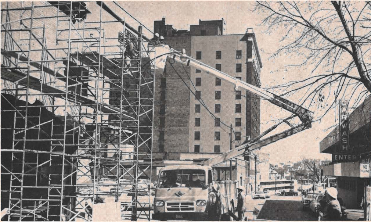
A Roanoke district line crew helped out in the construction of the addition to the general office building there. To permit the erection of steel scaffolding for use of bricklayers, a 4-kv line had to be covered with fiber duct and moved away from the building. D. R. Hunt's crew did the job.
