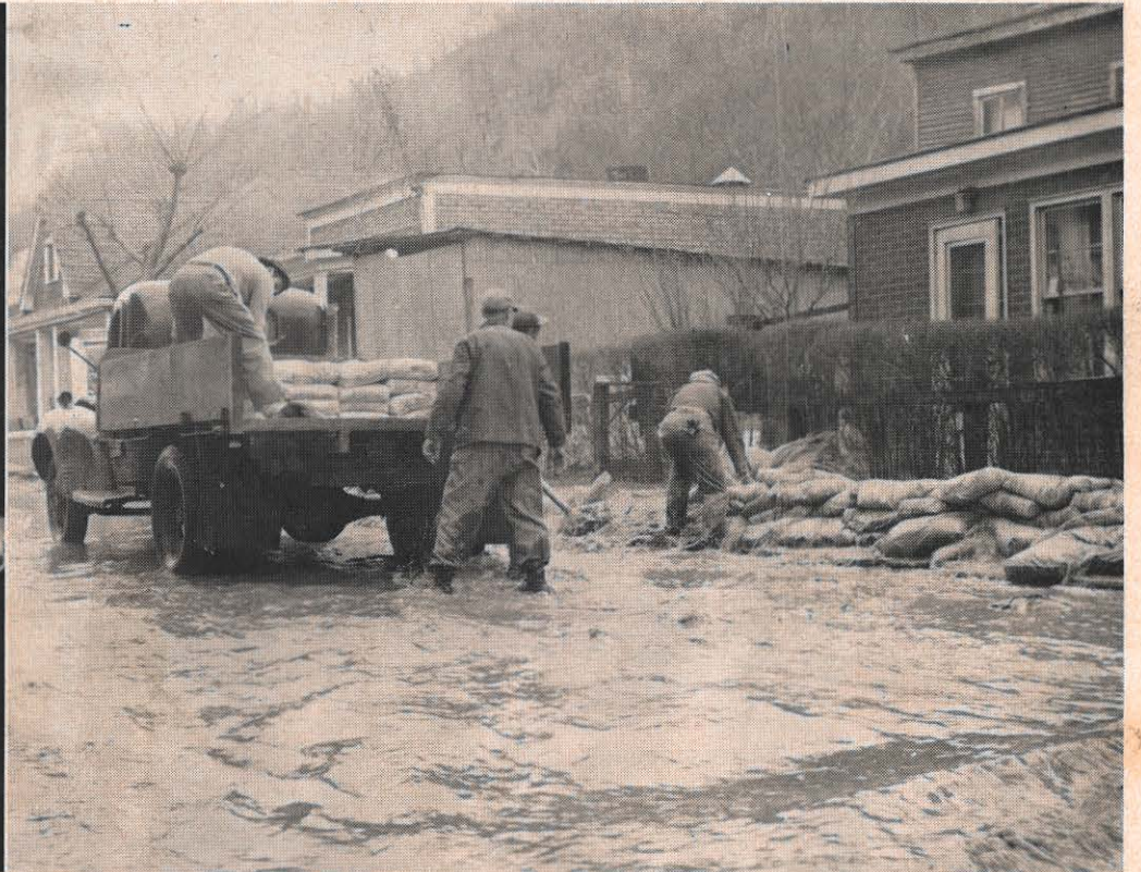
Exemplifying the fight put up by residents of the four states suffering from flooding were these citizens of Williamson. They are shown working feverishly to plug a break in the sandbag installation on Williamson's First Avenue above the floodwall. Although there was seepage, the sandbags did a good job of preventing heavy flooding, joining the town's floodwall in the battle. Photo courtesy Williamson Daily News. Other pictures of the flood can be found on pages 6 and 7.
