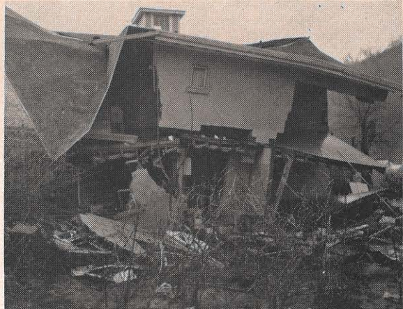
The wreckage of this apartment house on Cline Street in Pikeville was left behind by the record flood hitting that city.
