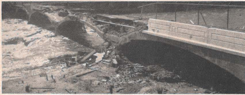
At top, water inundates Pikeville High School at left, while at bottom receding water leaves the wreckage of a school bridge at Pineville.
