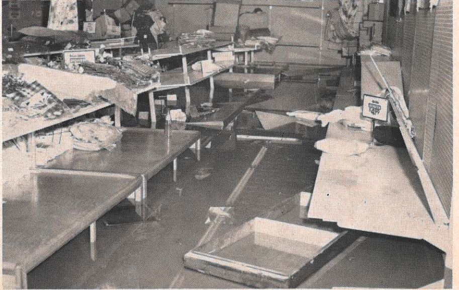
Deserted except for rising water is the basement of Watson's Store on McDowell Street in Welch.
