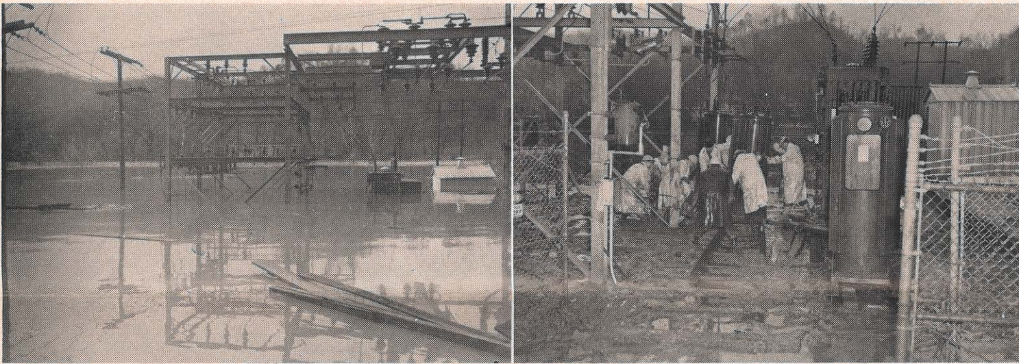
Pikeville station was hard hit. At left, this is what the yard looked like four hours before the water crested. At right, a mud-covered crew replaces a burned-out regulator at the station after the water has receded.
