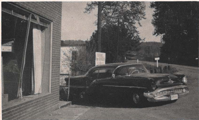
In the first four and a half months of the year, no less than eleven distribution poles have been broken off by motorists in the Fieldale district, each smash coming on a weekend. In the latest accident, the damage came closer to home: a car crashed into the Fieldale office building, breaking the display window and damaging the auditorium wall.
