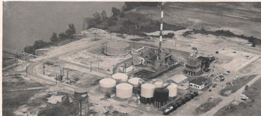
Making important contributions to the economy of the Ashland area are these plants of an older industry and a newer one. A stalwart in the economy is the Greenup plant of E. I. Du-
