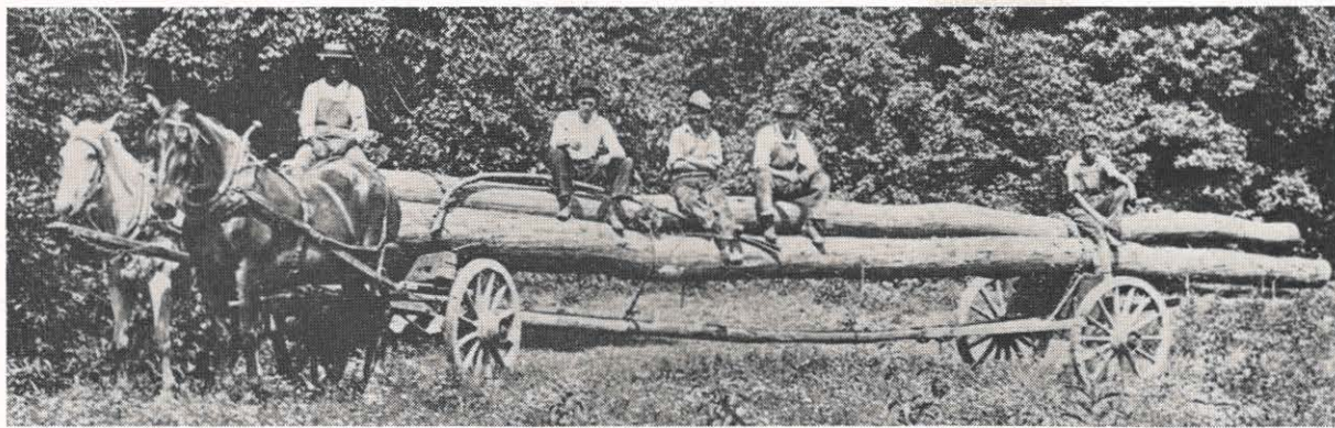
Helping get the line-building job done back in 1908 was this horse-drawn pole carrier. This crew is carrying chestnut poles for the old Kanawha Water and Light Company in Charleston.
