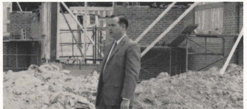
Clyde Marshall, Beckley records supervisor, stands in front of the Lutheran Church now under construction in Beckley. He was a member when services were held in the Appalachian auditorium, is a trustee, a member of the building committee, and no doubt helped make the decision to make it the first total electric church in Beckley.
