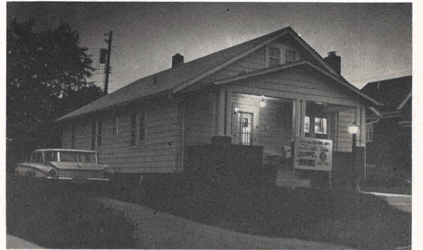
A 30-year-old house, like thousands in our service area, was taken over by the Ashland Academy of Lighting Arts for remodeling, and the result is a perfect glimpse of what an older home can be turned into by going Total Electric.
