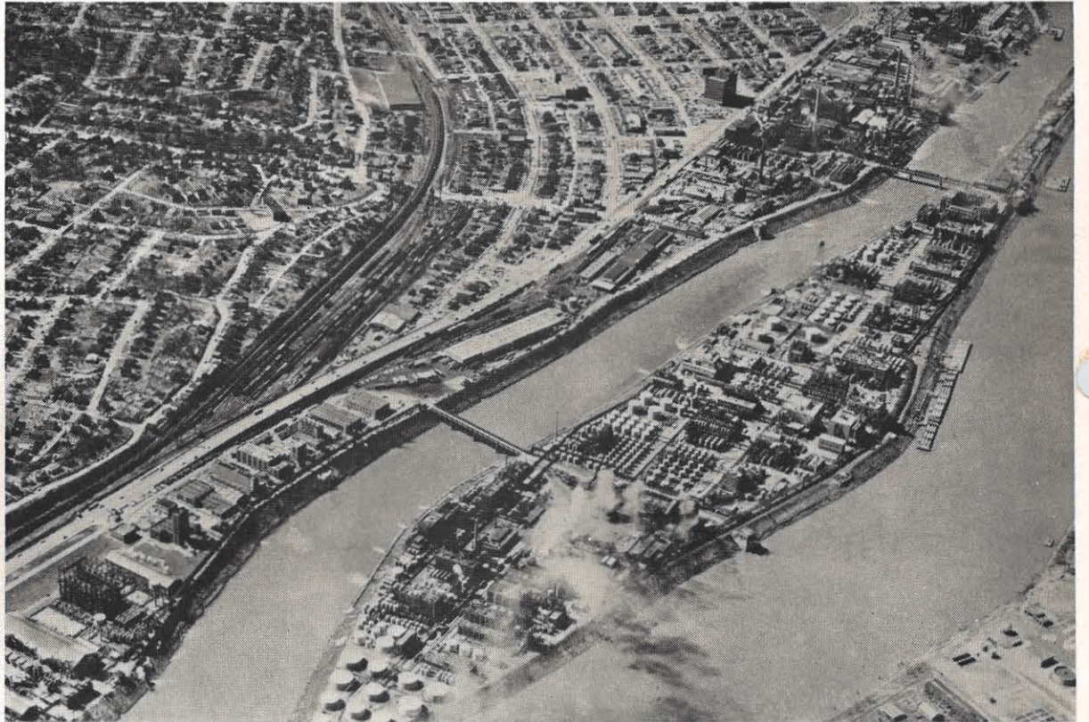
Union Carbide has made the most of land in South Charleston, bridging the Kanawha River to expand its facilities onto Blaine Island. The island is often referred to as an "industrial battleship."
